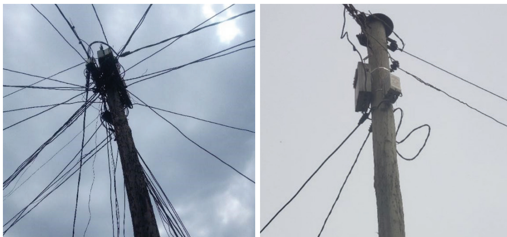
Photo caption: Comparison of the number of prepaid meters and wires dropping down from a utility pole. One pole shows the ideal of two prepaid meters and two service lines (left) while the other features few meters but many service lines originating from the same pole (right). Photos provided by YouthMappers.
