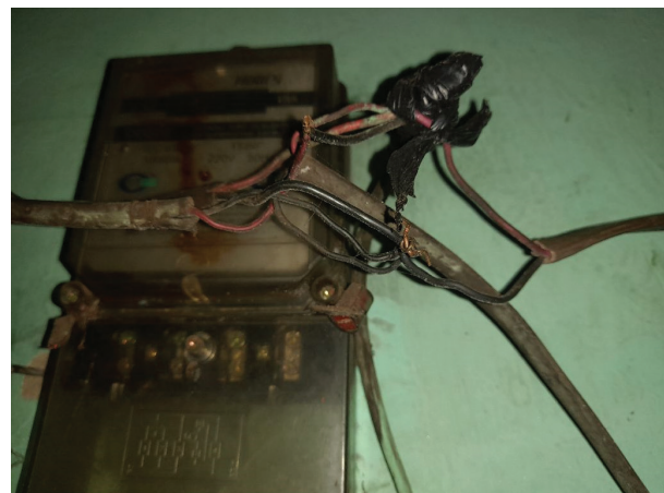
Photo caption: Wires which are improperly spliced and bare, which are at risk of transferring current into materials or people who come into contact with them. Photos by Paul Kyoma.
