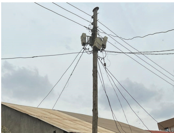
Photo caption: Example of mapped utility pole with white boxes which are prepaid meters on the pole and service lines dropping from the pole to houses. Photo provided by YouthMappers.
