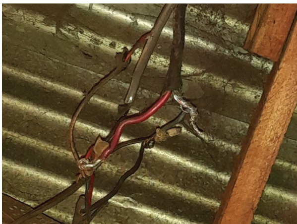
Photo caption: Wires which are improperly spliced and bare, which are at risk of transferring current into materials or people who come into contact with them. Photos by Paul Kyoma.
