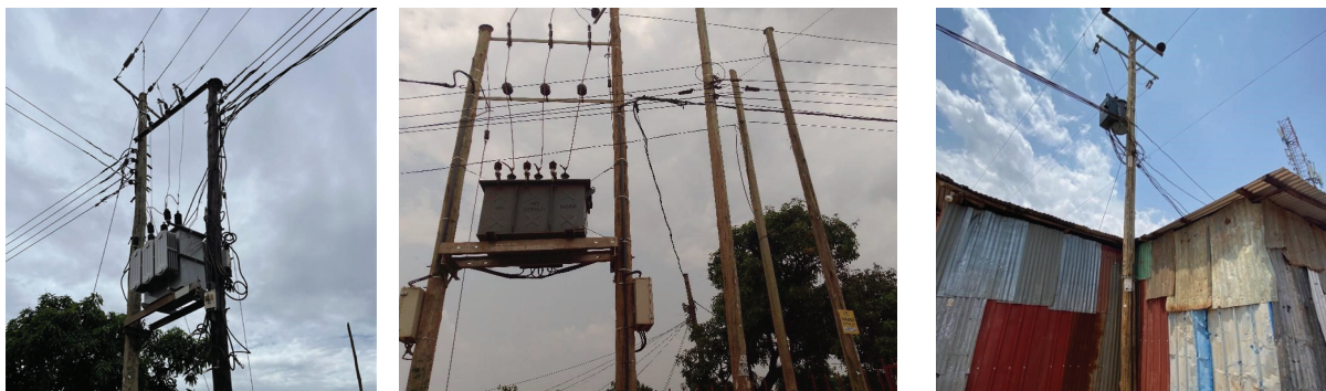
Photo caption: Three types of mapped transformers. Two high capacity and one low capacity transformers. Photos provided by YouthMappers and Elena van Hove.
